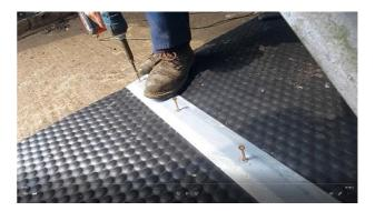
Make sure that the <u>sleeve of the frame fixing is in contact with the strip and the head of the screw</u> as this helps to prevent corrosion
