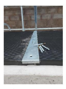
It is of CRITICAL IMPORTANCE that you drill the hole deep enough for the fixing to tighten into the Mattress leaving no protrusions.
