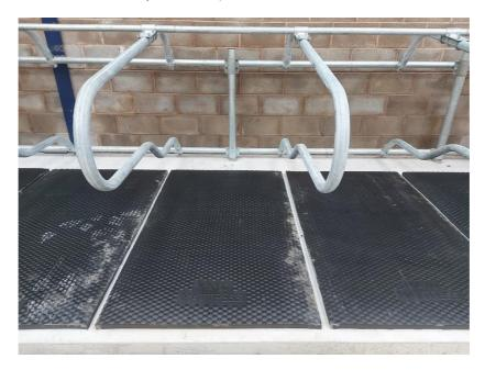
If you have legs in the bed (Mushroom / Newton Rigg style cubicles) Then the mats are right-sized **fitting in between the legs**. There is no need to cut notches for the legs See below:
