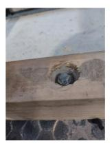
**TIP:** Screw the excess of thread so the nut has just tensioned the sleeve bolt and **no more for sleeve anchor bolt.**
