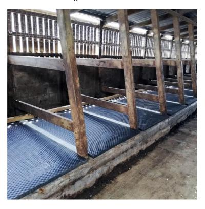
**Method detail**: Simply cut a notch for the mattress to sit around the leg of the kennel leaving 5mm (to allow the joining strip to fit at the back of the leg)
