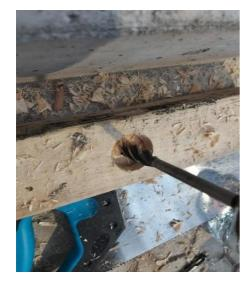
Put in 16mm Augur/Wood bit and drill through to the ground. If using Thunder bolts & Washers, use 12mm bit.
